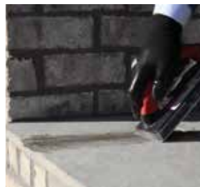
PIC 1. Fill joint with grout.
