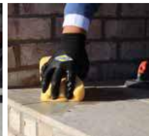
PIC 2. Remove excess grout with clean water.
